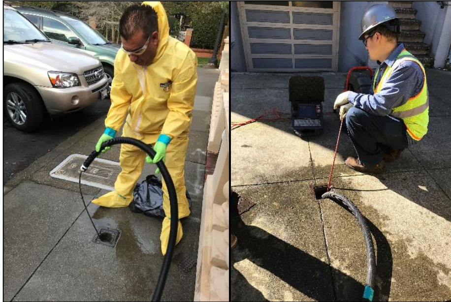
Figure 13 (left-right)— Plumber’s snake modification to the hose to assist with p-trap navigation. Water extraction and camera inspection occurring simultaneously at a multi-family complex.
